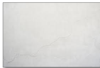
Hairline Cracks
